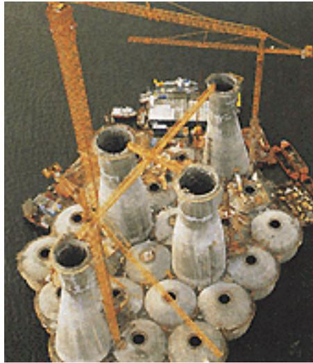
The post accident investigation traced the error to inaccurate finite element approximation of the linear elastic model of the tricell (using the popular finite element program NASTRAN).
