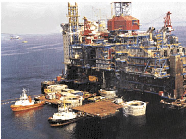
deck weighs 57,000 tons, and provides accommodation for about 200 people and support for drilling equipment weighing about 40,000 tons. When the first model sank in August 1991, the
