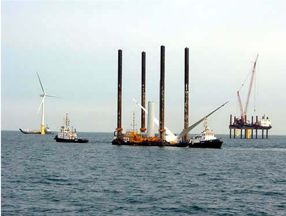
The Mayflower Resolution during installation of turbines at the North Hoyle offshore wind farm.
