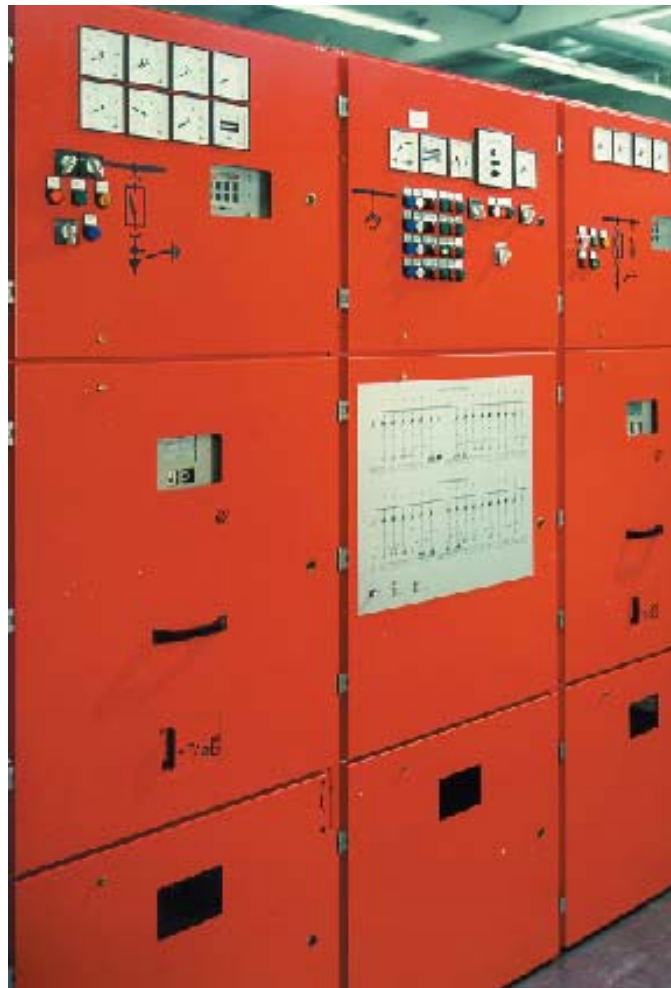
Switchboard: 10 kV High Voltage
