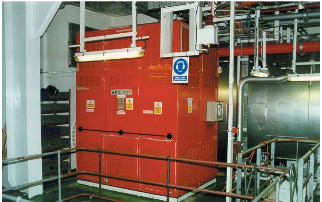
Propulsion transformer
