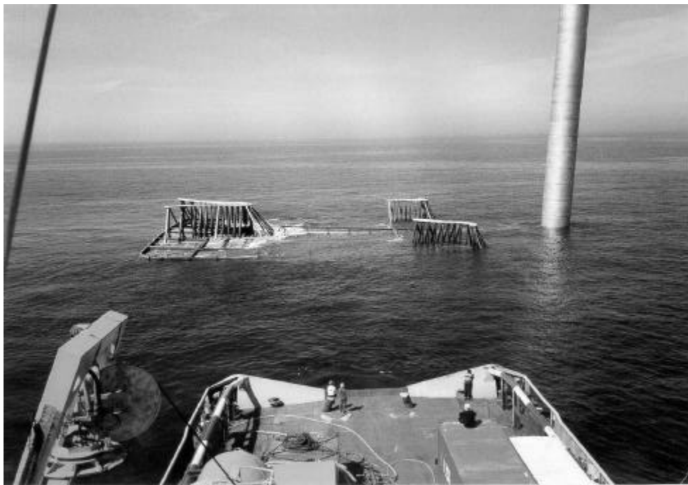
Figure 11: Roof of tank being submerged
