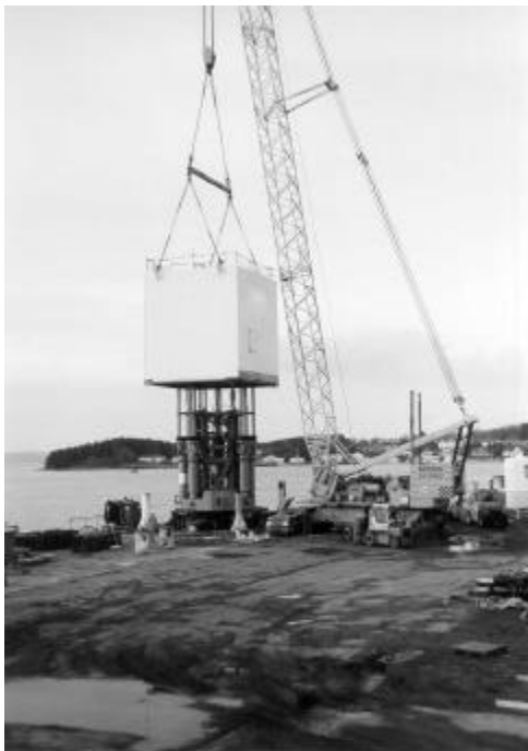
Figure 7: Assembly jacking system in jack house
