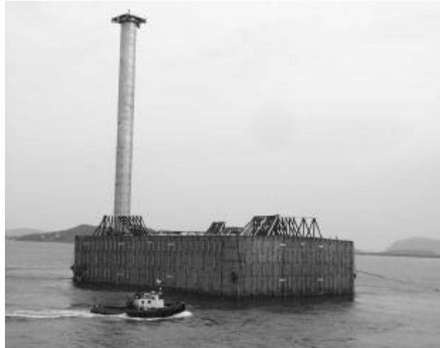
Figure 10: Wet tow of tank
