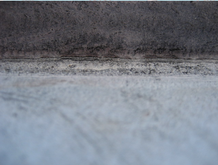
Surface Longitudinal Crack
