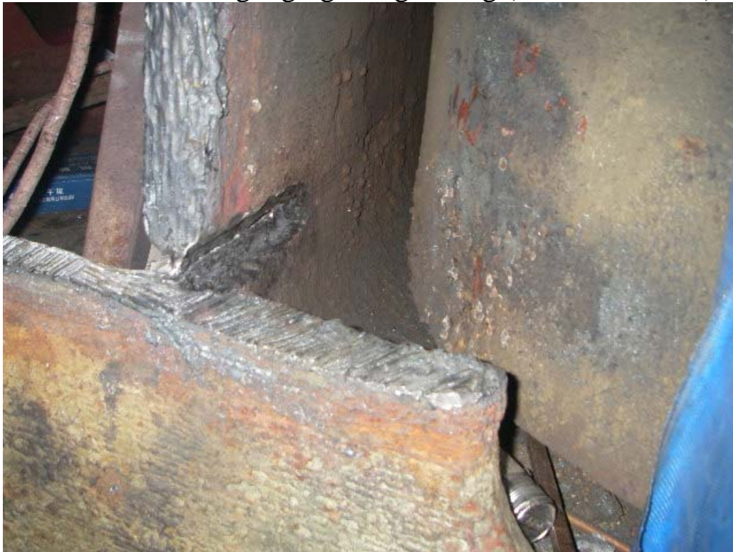
Crack in web after gouging and grinding (from both sides)
