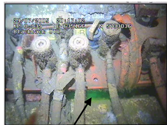
Control Fluid Leak from Subsea Umbilical Termination Assembly
