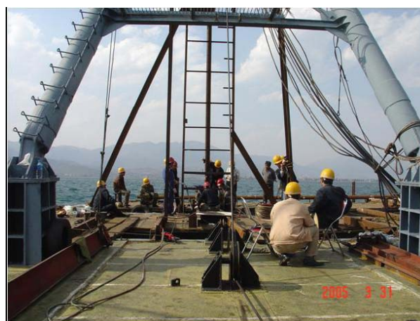
Fig. 4 Situation of the test of deepwater drilling in a lake of Kunming, China
