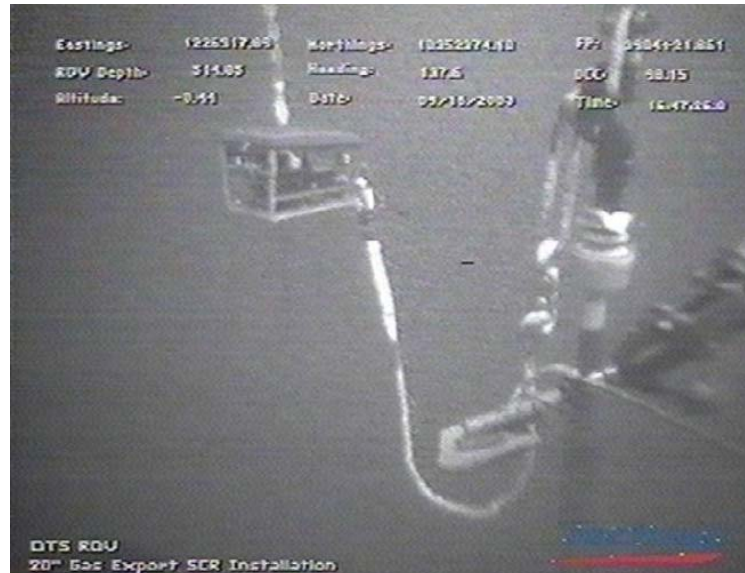
Figure 10 ROV deployed Synthetic Sling Riser Transfer Rigging
