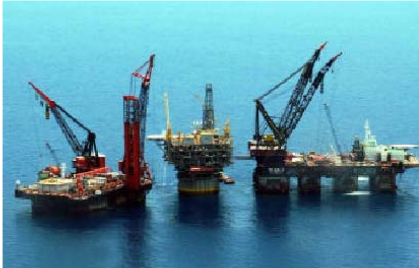
Figure 11 Spar under Construction
