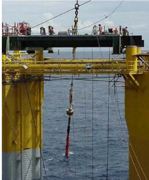
Figure 6 The Prince SCR during Hang-Off Installation showing the Pre-Installed VIV Strakes
