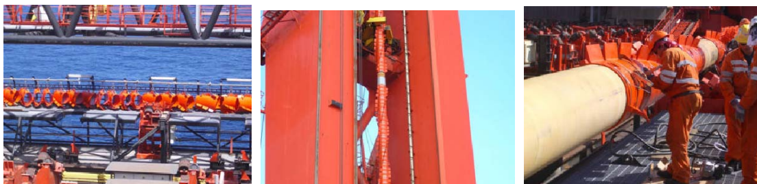
Figure 12 a: VIV suppression strake installation platform; b: Pre-installed strake area; c: Strap installation
