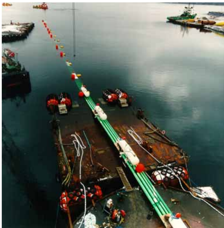
Figure 6-6: Riser Bundle System at Launch Operation
